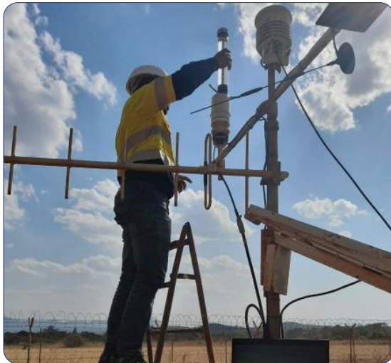
Installation & calibration of Weather Station
